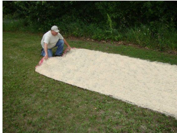
Figure 4. Properly position unrolled RECP for installation.
