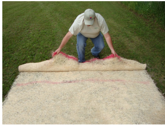
Figure 2. Pull end of RECP along red line.
