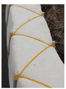
**Step 5** Backfill to the top of the Curlex Blocs. If desired, seed and fertilize backfill area. Install Curlex<sup>®</sup> NetFree<sup>™</sup> onto the backfill area. If desired, plug plants through the Curlex NetFree.
