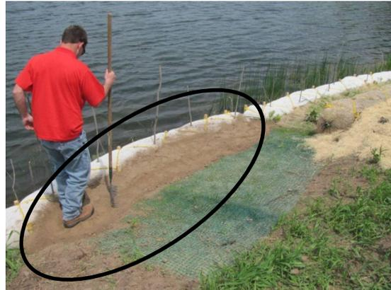
**Step 6** If desired, use a planting iron to create a pilot hole through the Bloc. Insert a live stake through the pilot hole into the subgrade a minimum of 6 inches below the Bloc.
