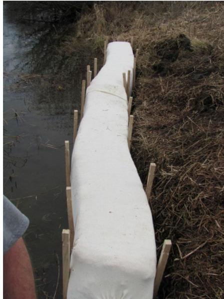
**Step 4** Weave rope from stake-to-stake, front-to-back along the length of the Blocs. Drive the stakes the remaining 3-4 inches or until the rope is tight.
