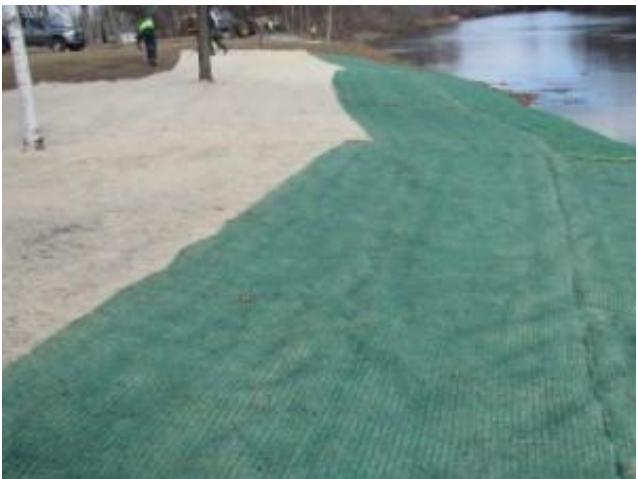
Heavy Duty Curlex Blankets, for long-term protection against wind and water erosion, are a natural choice in place of stone or riprap in swales, ditch bottoms, and on long, steep slopes.
