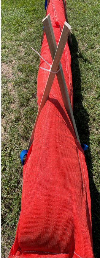
Criss-crossed staking installation.
